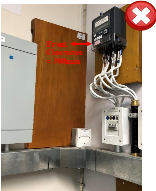
Front clearance of the wooden board less than 900mm is not allowed.
